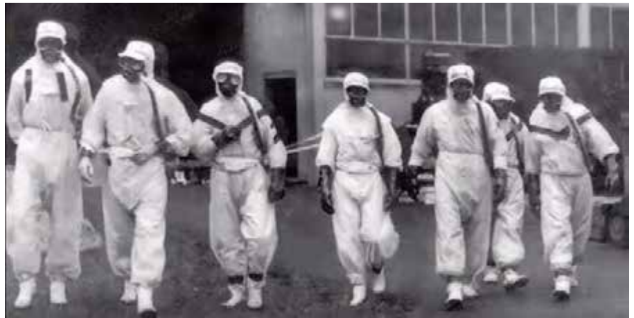
Workers at the Windscale nuclear power station tackle the fire in 1957. The plant was subsequently rebranded as Sellafield. (Image: 'Windscale: The Story of Britain's Chernobyl' / Fascinating Horror / YouTube)
